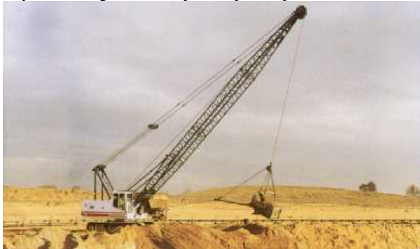
Figure 3. Dragline (crane) excavator in operation.
