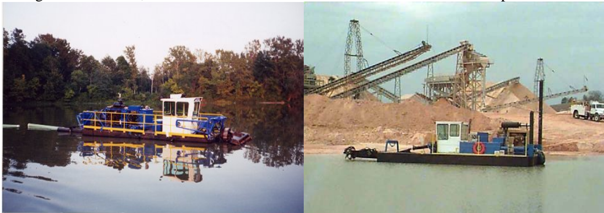
Figure 5 and 6. Photographs of hydraulic dredges showing two types of cutter heads.
